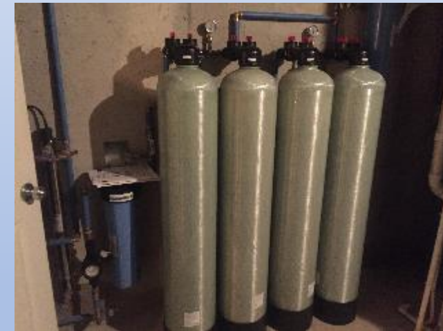
Photo: Example of a POE system installed by Wolverine
